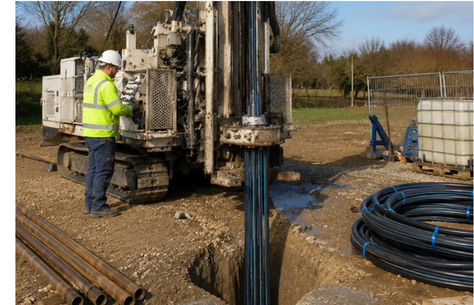
03 Vertical Ground Heat Exchangers
