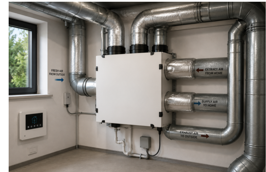
06 Mechanical Ventilation with Heat Recovery
