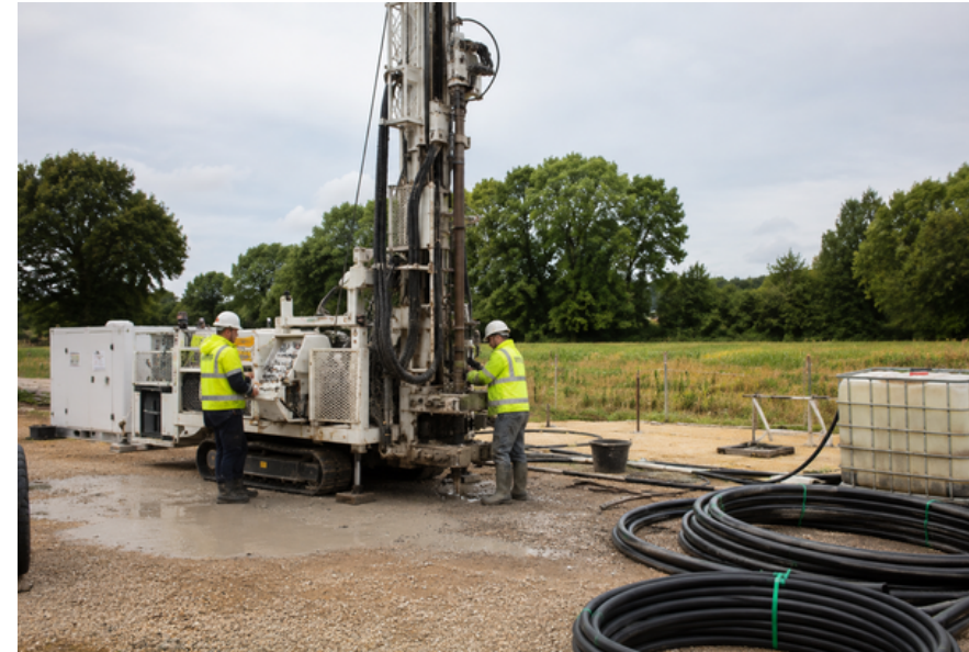
02 Vertical Closed Loop Boreholes
